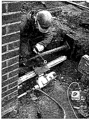
Diamond coring in process below ground level through masonry.
