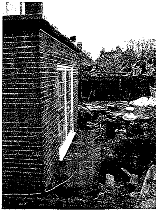
Extension to be stabilised
