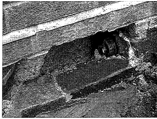
Tendon located within cored duct and dead anchor plate positioned.
