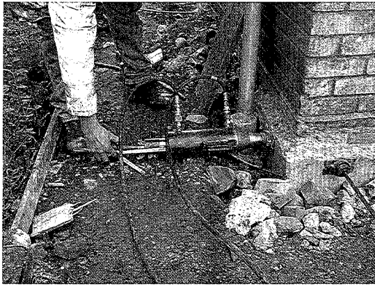
Post tensioning in progress.
