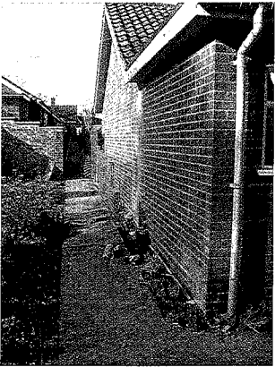
Installation in progress, note lack of disruption.
