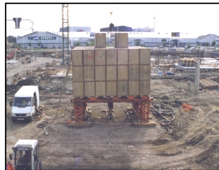
Static load testing
