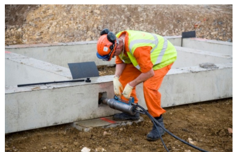
Post tensioning the system
