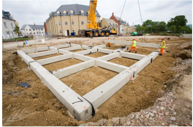
Lifting the beams into place
