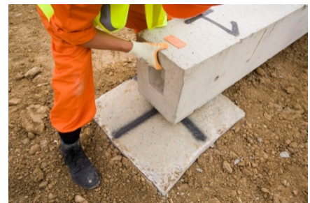
Aligning the beams
