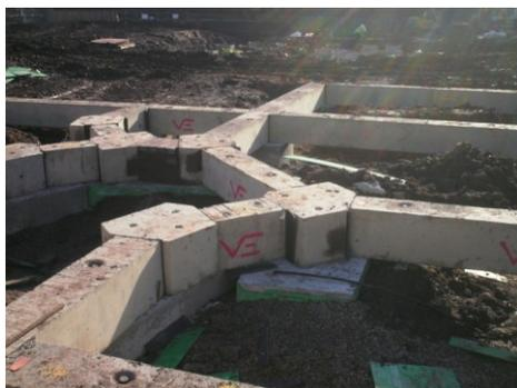
As Smartfoot® precast modular foundations are completely bespoke, they aren't limited to typical angles.
