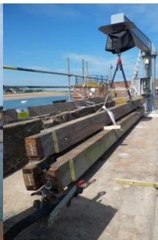
The new crane being used to lift a stop log into position.
