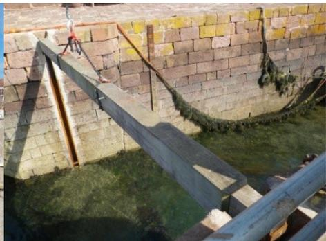
The first stop log being lowered into position in the stop log channels.
