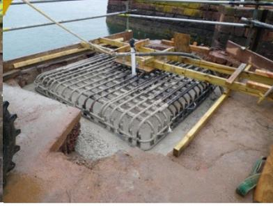
The steel reinforcement for the foundation of the new pier crane.
