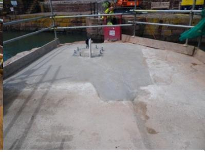
The new pier crane foundation having been concreted and awaiting the arrival of the crane itself.
