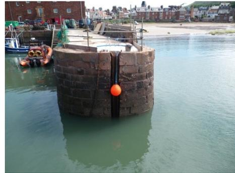
Right: One of the completed stop log channels installed at the end of the pier roundhead.
