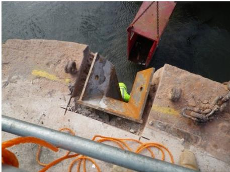
Left: One of the two stop log channels being checked prior to being grouted into position.
