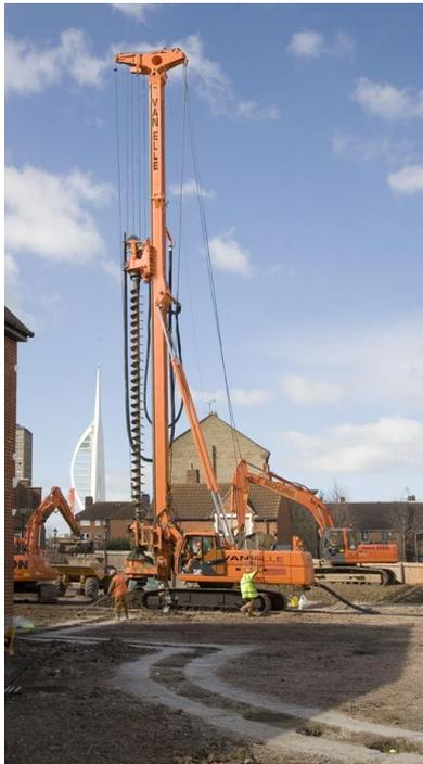
From the initial design to the completion of the project we consulted with the client on a regular basis, designed the wall to meet their construction programme, constructed a guide wall, installed all the bearing piles and piled the secant wall.
