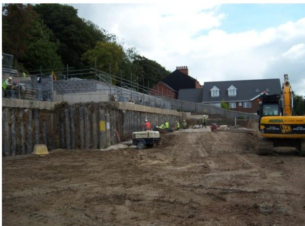
We also installed 30No. 450mm diameter, 9m deep piles adjacent to the driveway of the house to the east of Carline road. This was to retain the driveway and property when the steps were excavated.
