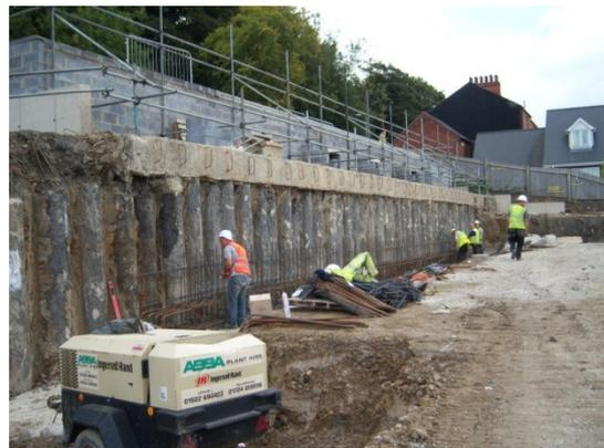
Installing steel at the base of the retaining wall
