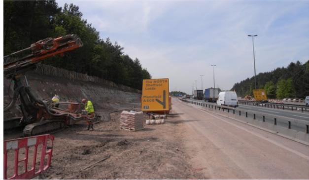
Van Elle installing soil nails to stabilise the embankments.
