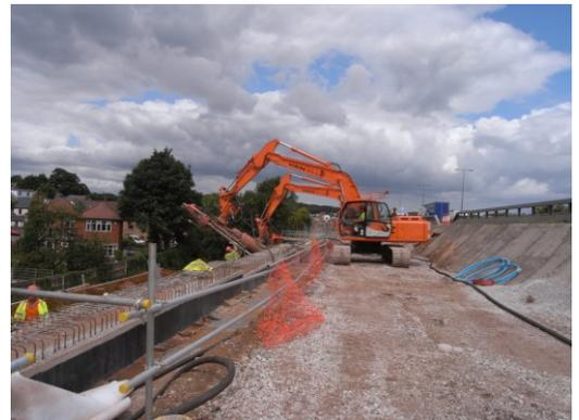
Van Elle installing anchors to the piled retaining walls using new innovative rigs.
