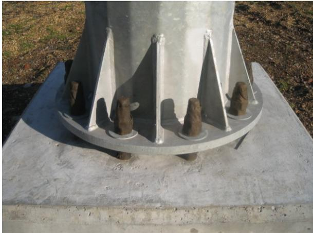
The plinth and anchor bolts for a high mast column.
