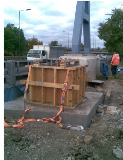
A column base being cast next to the A52 post-piling.
