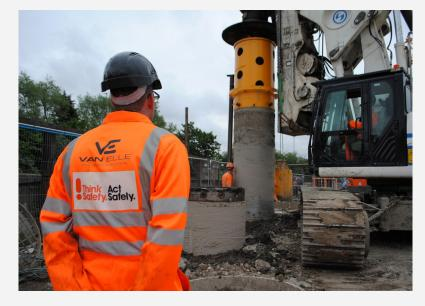
Van Elle was selected by main contractor Jackson Civil Engineering to install a hard-hard secant wall on a river wall replacement scheme on Dormay Street in London. This particular solution was chosen in order to meet the requirements of the 65-year lifespan requested by the client..
