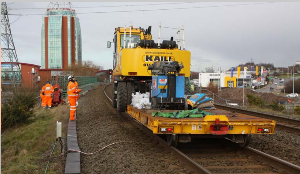
RRV towing the plant and materials on a trailer
