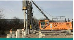
Junttan PM20 installing pre-cast driven piles
