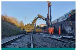
Continuous Flight Auger (CFA) on track solutions
