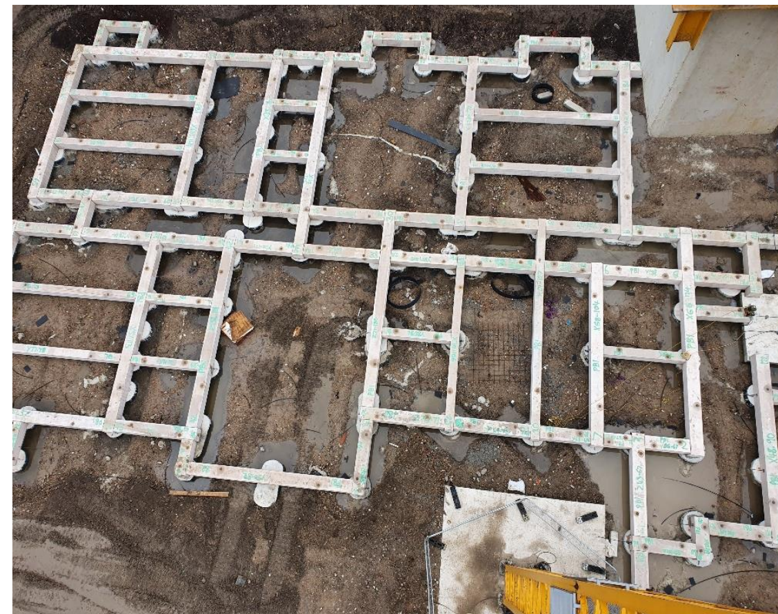
Smartfoot installation at Bingley, Yorkshire for McCarthy & Stone
