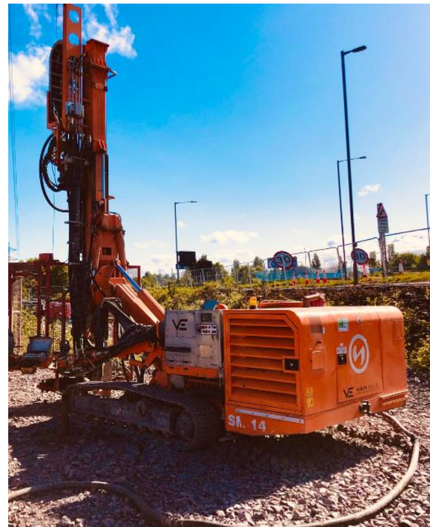
Drill & Grout to mine-workings at M6 junction 10, Walsall
