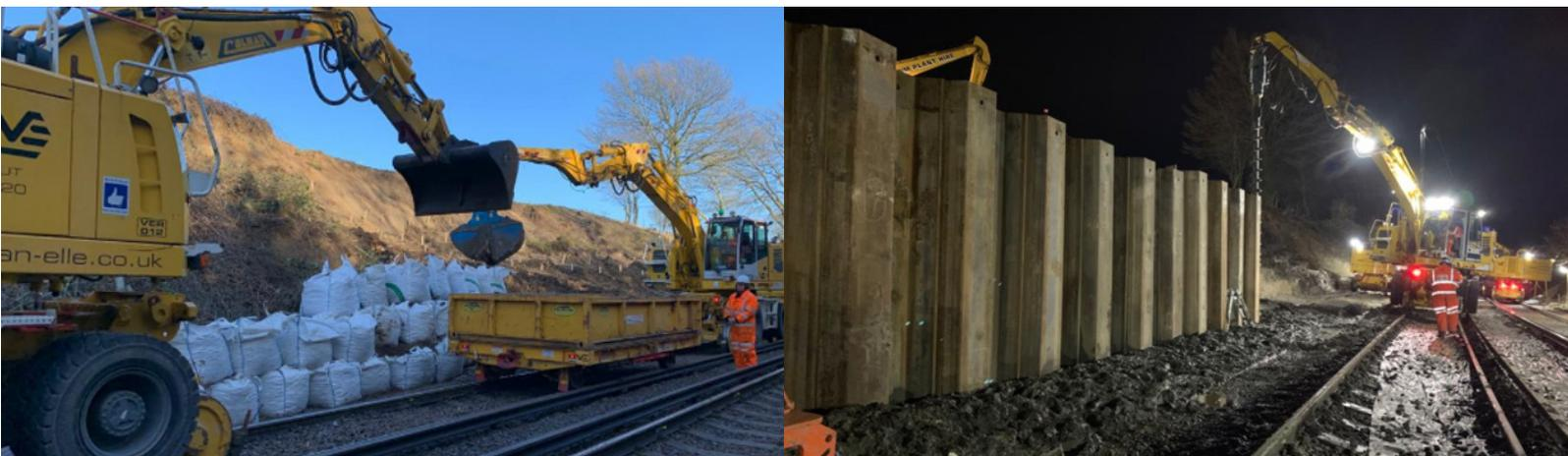
**From ground investigation and design, to the installation of a permanent retaining wall and rebuilding a failed embankment, our team worked around the clock to enable the quick re-opening of a railway line in the South East.**
