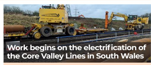
In July piling works started on the Core Valley Lines in preparation for the electrification of the South Wales Metro.
