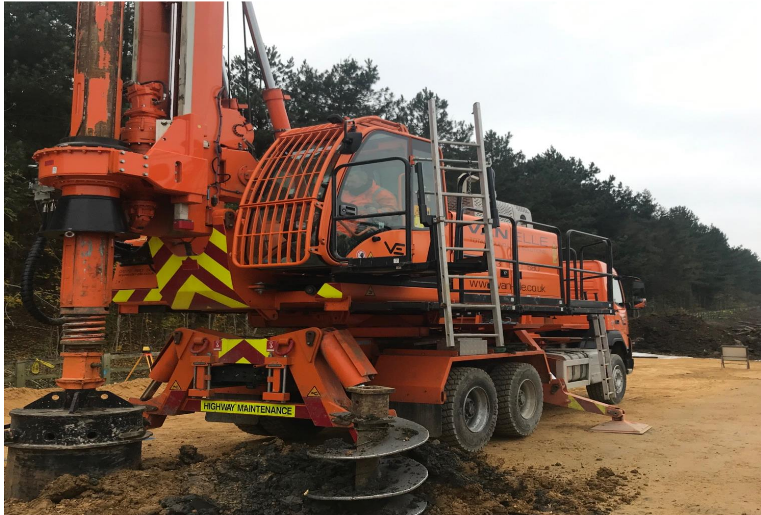
Both lorry-mounted rotary rigs were mobilised on the M1 in the period – key assets for our smart motorway strategy
