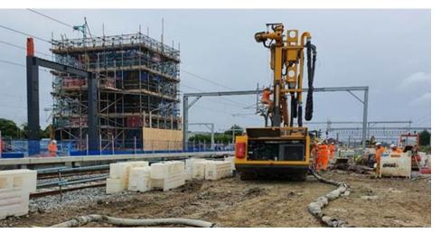
For our client Volker Fitzpatrick we recently completed both the on and offtrack piling works at the new Brent Cross West Station, London.
