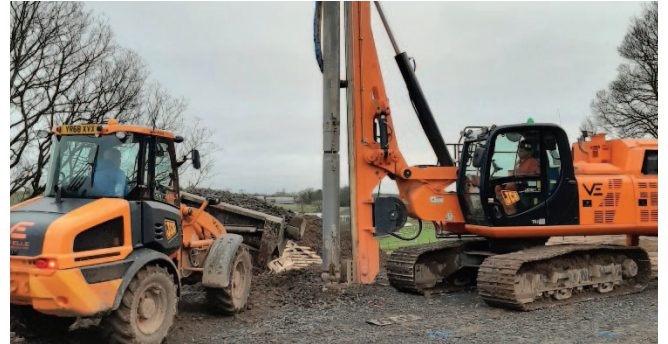
Vibro stone column installations for Cala Homes in Erskine, Scotland
