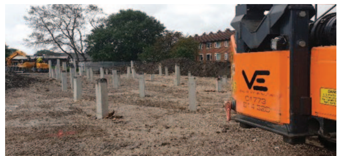
Smartfoot precast modular ground beam system to be installed on driven piles for modular home developer Ilke Homes.
