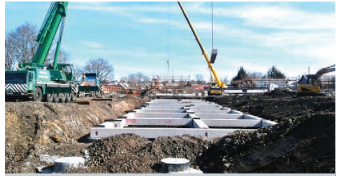
Smartfoot ground-beam system being installed by crane at Love Street, Scotland
