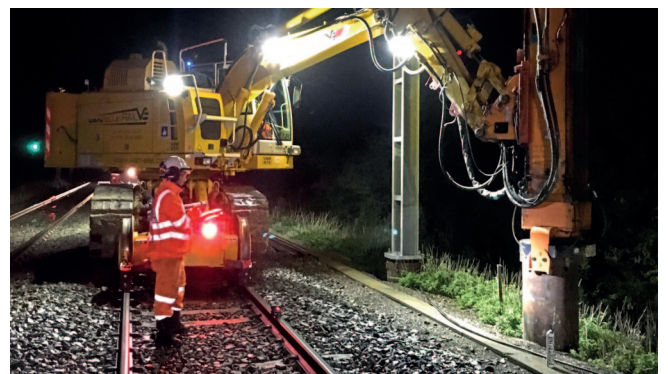
Van Elle install last pile for Midland Mainline Electrification on behalf of SPL
