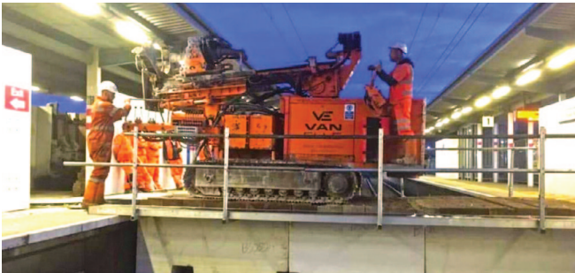
Luton Airport Parkway - new bridge foundations installed for AmcoGiffen
