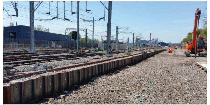
Old Oak Common - Lorclon/Taylor Woodrow Any Line Open (ALO) sheet pile installation for Crossrail carriage wash
