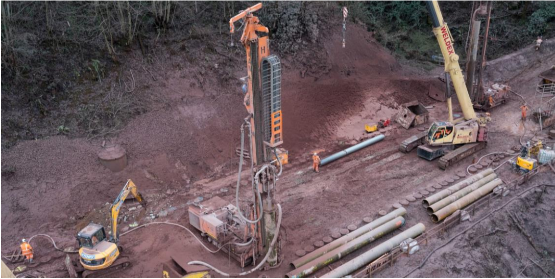
Eden Brows – stabilisation of a deep slip on Carlisle to Settle line FY19, c.£5m for Story
