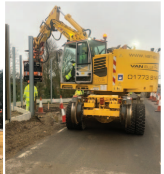
King Post installation on M4 jcn 3 to 12
