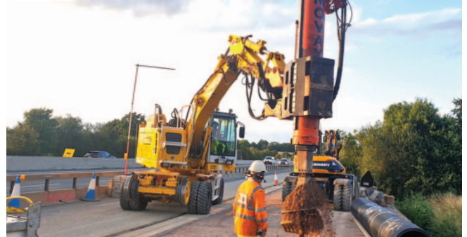
Minor structures installation on the M23 jcn 8 to 10
