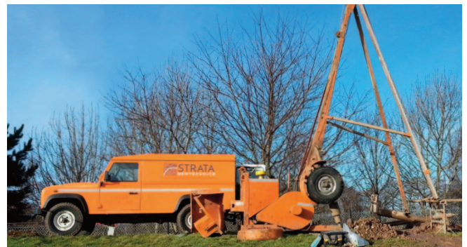
Ground investigation for the A428 Black Cat to Caxton route improvements
