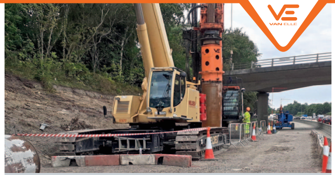
M27 jcn 4 to 11 Smart Motorway
