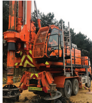
Lorry mounted rigs on the M1 jcn 13 to 16
