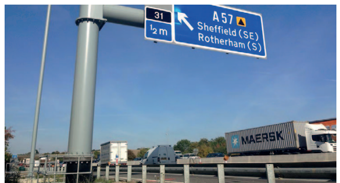
Helical piles and grillages on the M1
